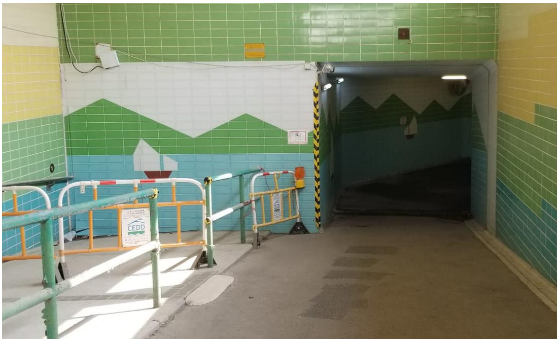
Photo 3 - Erection of site hoardings in unobtrusive colours
