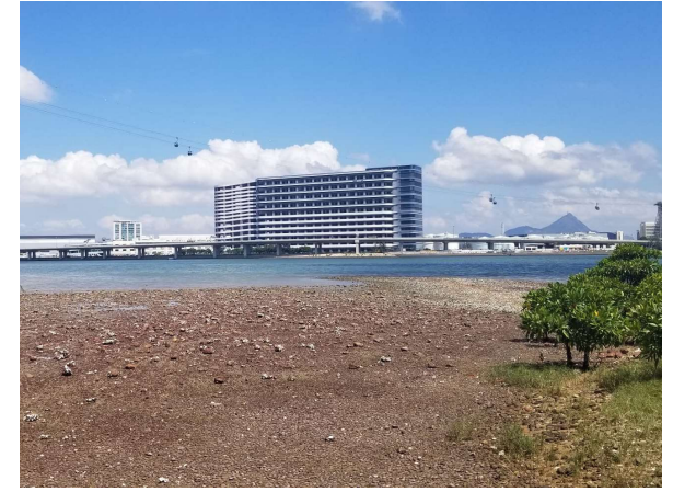
(c) Survey Location at TCB3
